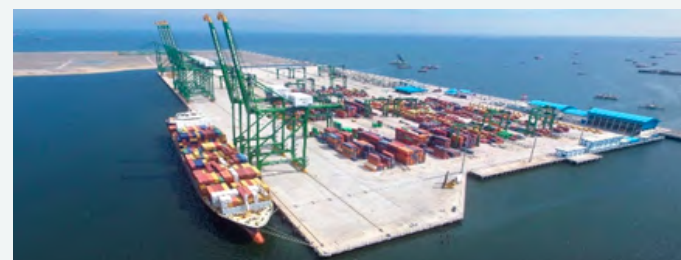
Royal Haskoning : Terminal contenedores Kalibará – Indonesia
